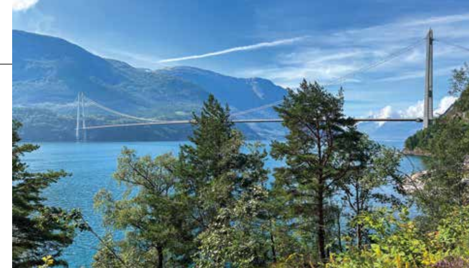
At 1,380 metres long, the Hardanger Bridge is the longest suspension bridge in Norway. You enter and exit each side via tunnels into the adjoining mountains.
