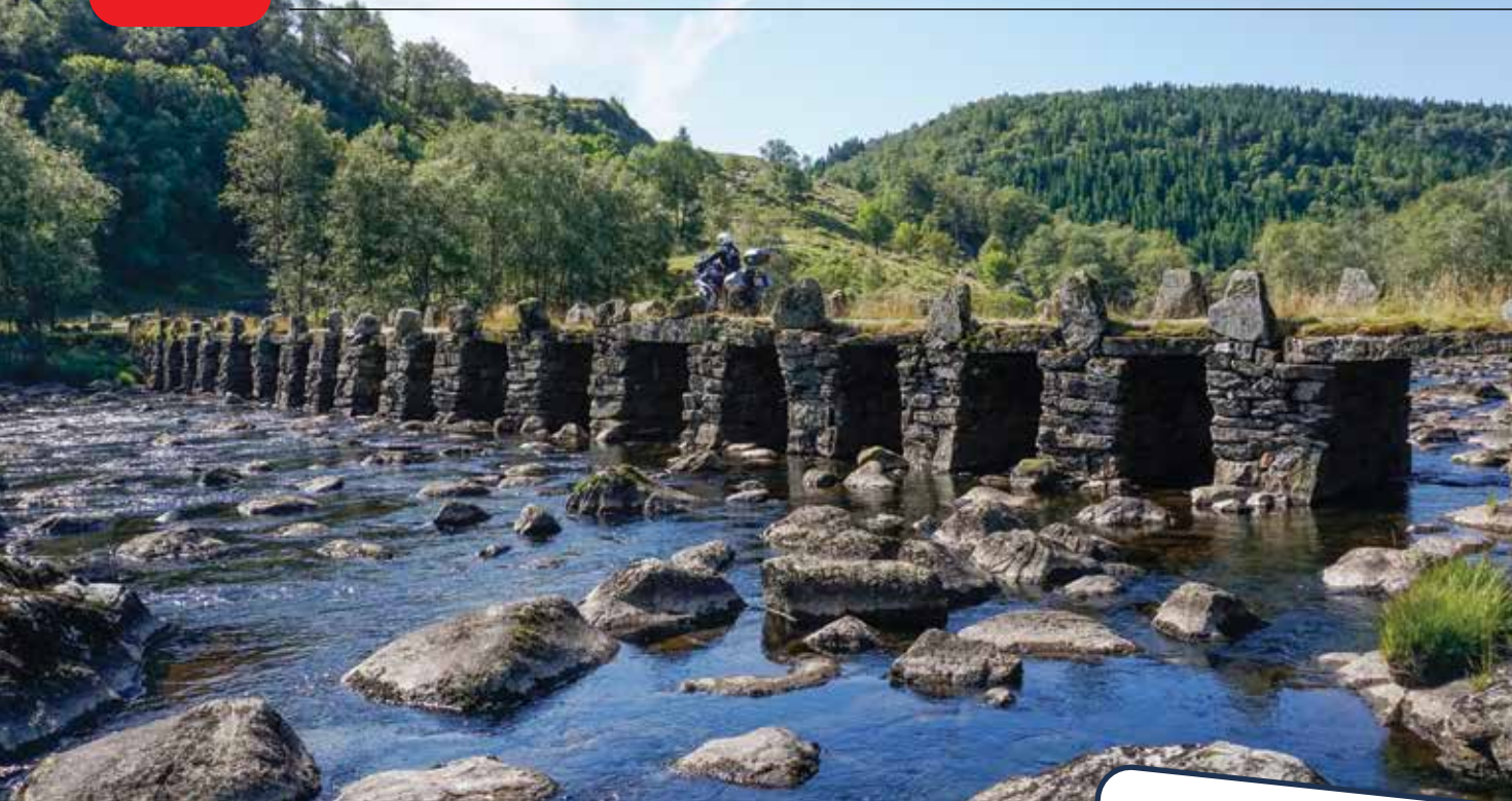
Built in the early 19th century, the Terland Klopp is a 60-metre-long dry-set stone slab bridge with 21 arches and is the longest and best preserved stone slab bridge in the Nordic countries. It was decommissioned in 1977.
